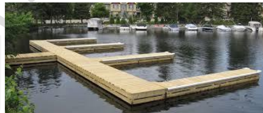
Figure 2.9: Floating dock based on Archimedes' principle
