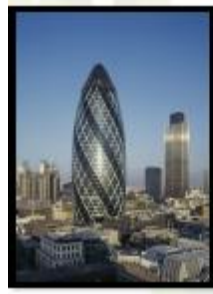
The Swiss Re Tower
